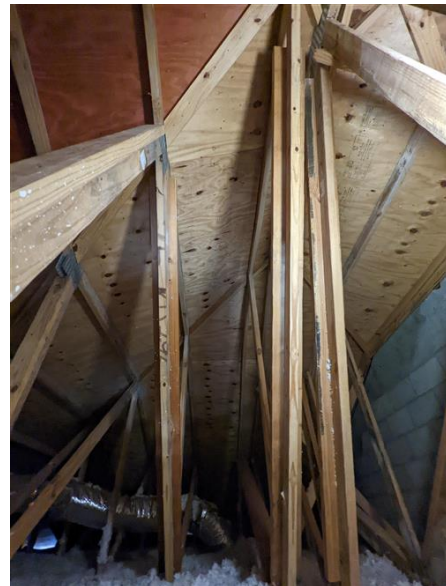
Underside Roof Deck
