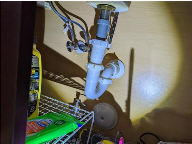
Bath Sink Plumbing
