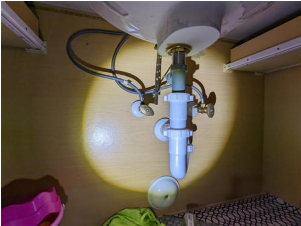
Bath Sink Plumbing
