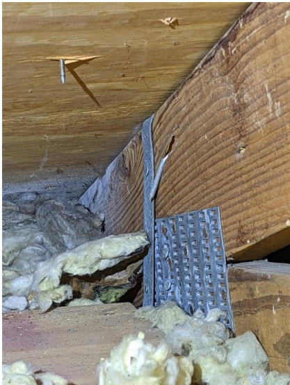
Wall to Roof Connection
