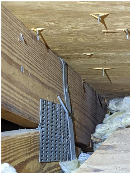
Wall to Roof Connection
