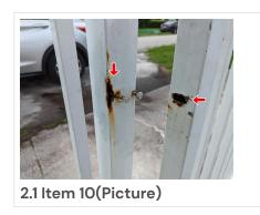
(4) Metal gate on left side of house does not close properly. Dead bolt does not line up with hole to lock gate.
